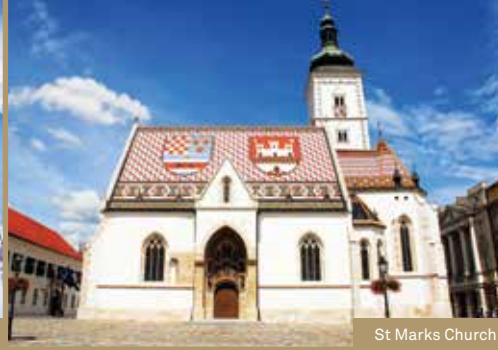
St Marks Church
